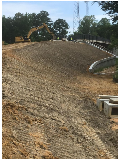
Photo: Crews grade slopes and place topsoil to accommodate the new roadway approaching the bridges.
