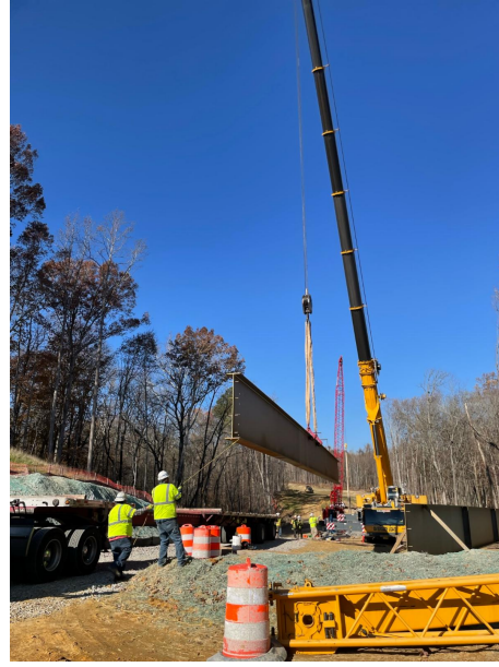
Photo: The first of the horizontal steel beams is delivered and placed on the Skiffes Creek Bridge.
