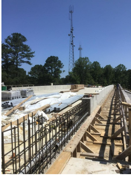
Photo: Concrete railings are constructed on the bridge over Route 143 and CSX rail as part of the final elements of the bridge construction.
