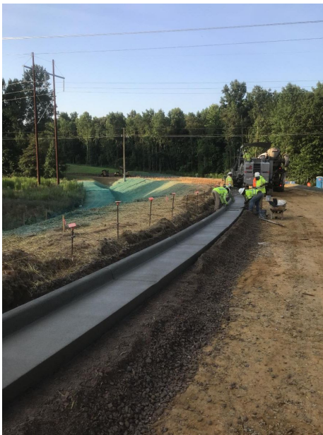
Photo: Crews work on the concrete curb and gutter for the approach roadway to Skiffes Creek Bridge.
