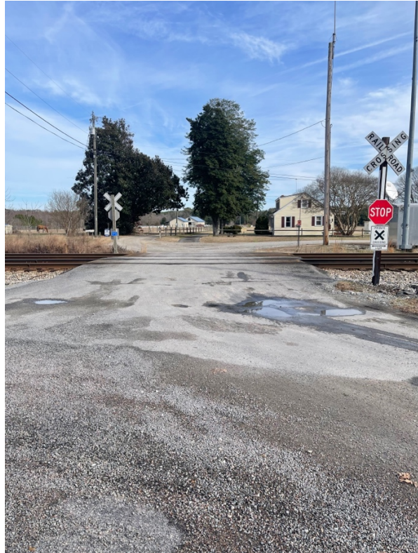
Head on view of Peach St CSX Crossing
